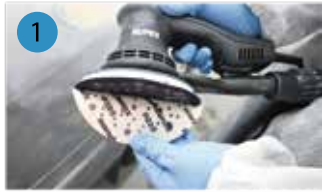
1 Repaired Area Sanding
